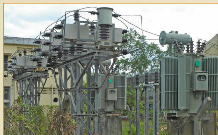
Outdoor Harmonic Filter Capacitor Bank
